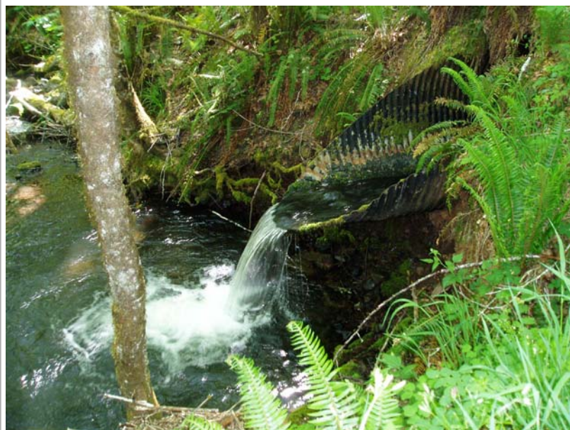
Perched culvert, a barrier to fish, where Stilson Creek joins Rock Cr.
